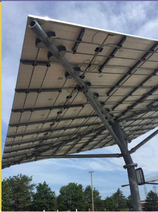
Photo: Bridgeview Courthouse Solar Installation
