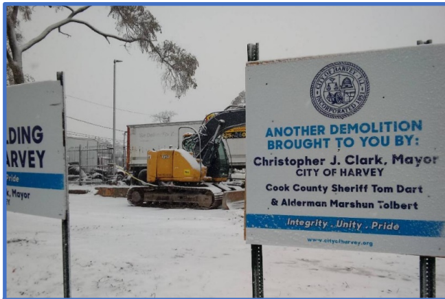
RENEW demolition site in Harvey
