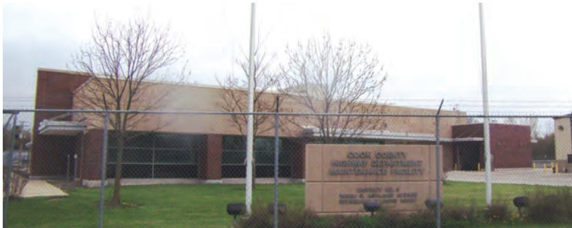
CCHD Maintenance Facility: District 5
