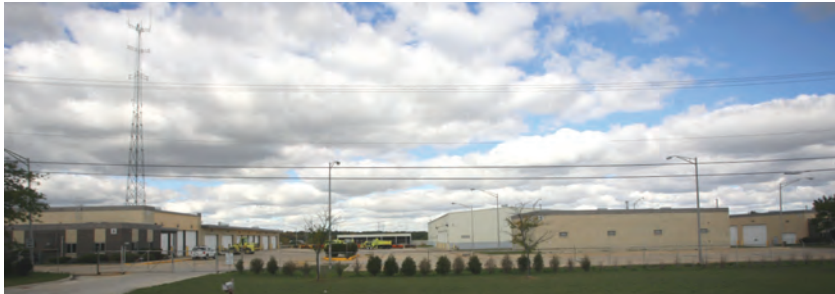
CCHD Maintenance Facility: District 4
