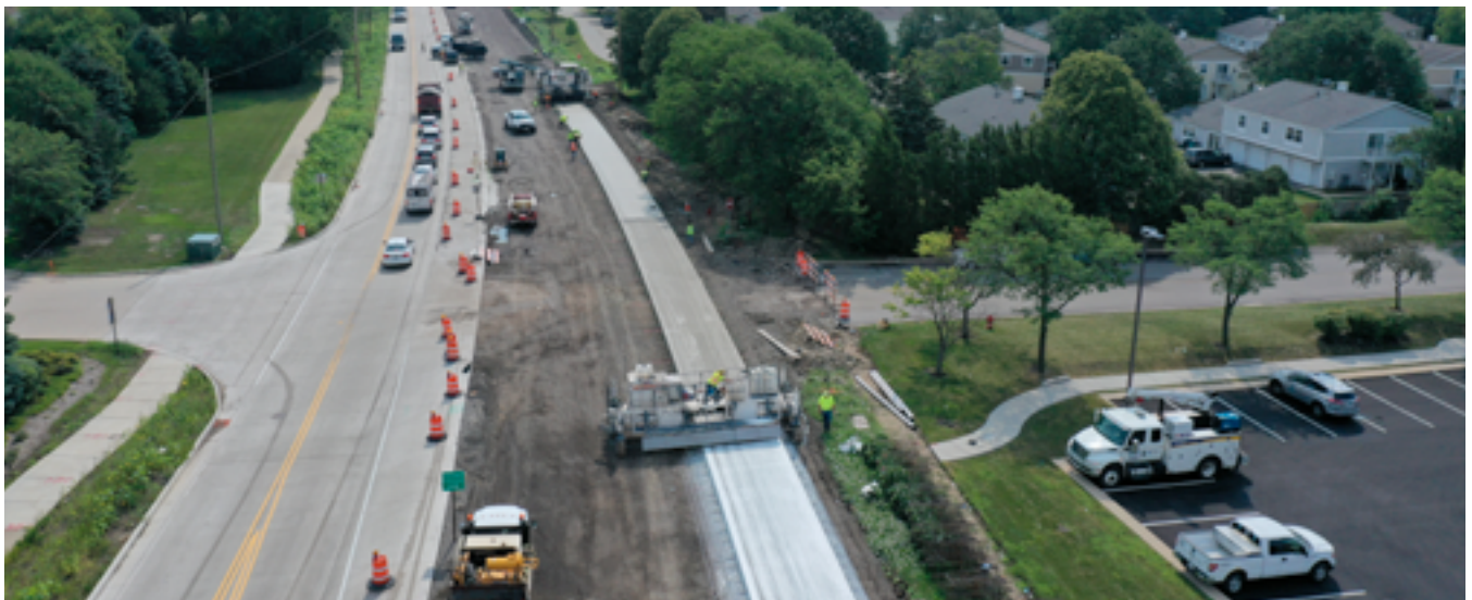
Figure 3: Construction on Lake Cook Road from Raupp Boulevard to Hastings Lane will be completed in FY2021.
