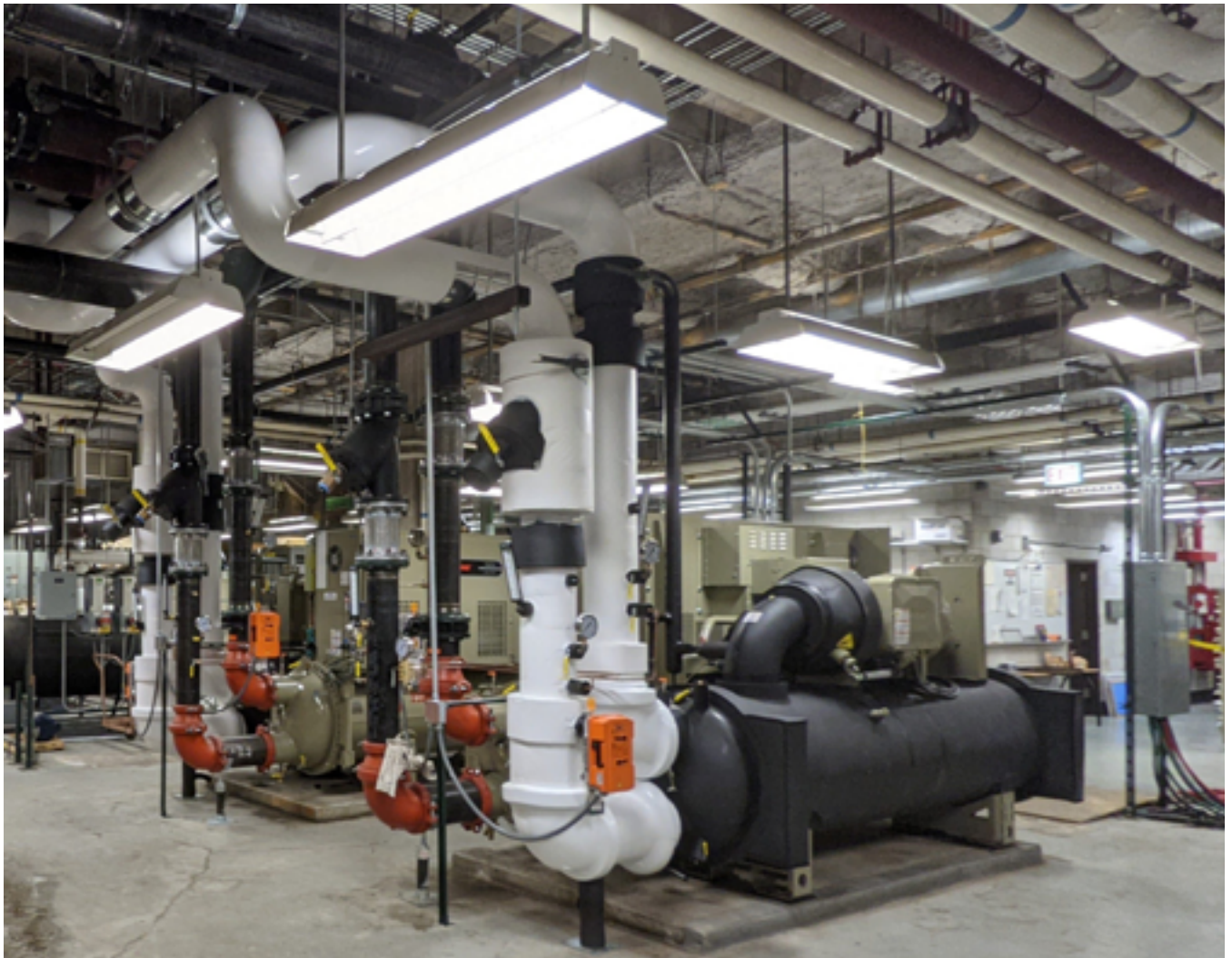
New energy efficient chillers at the Institute of Forensic Medicine
