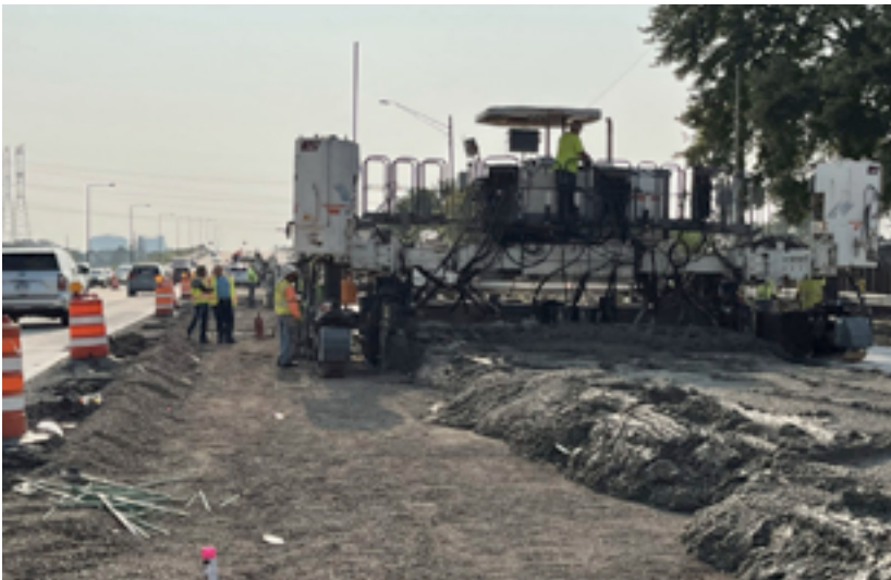
Figure 9: Cook County maintenance crews repair and maintain asphalt pavement surfaces. Existing surface was removed by milling, full depth deteriorated pavement areas were removed, patched with concrete and roadway overlaid with a new asphalt surface.
