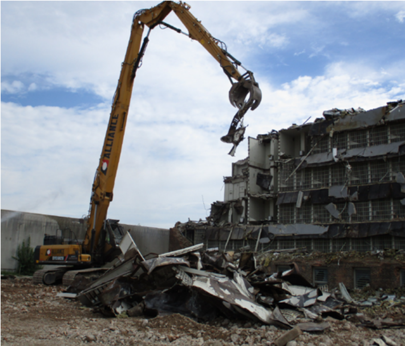
Demolition of Divisions I & IA at the Department of Corrections campus
