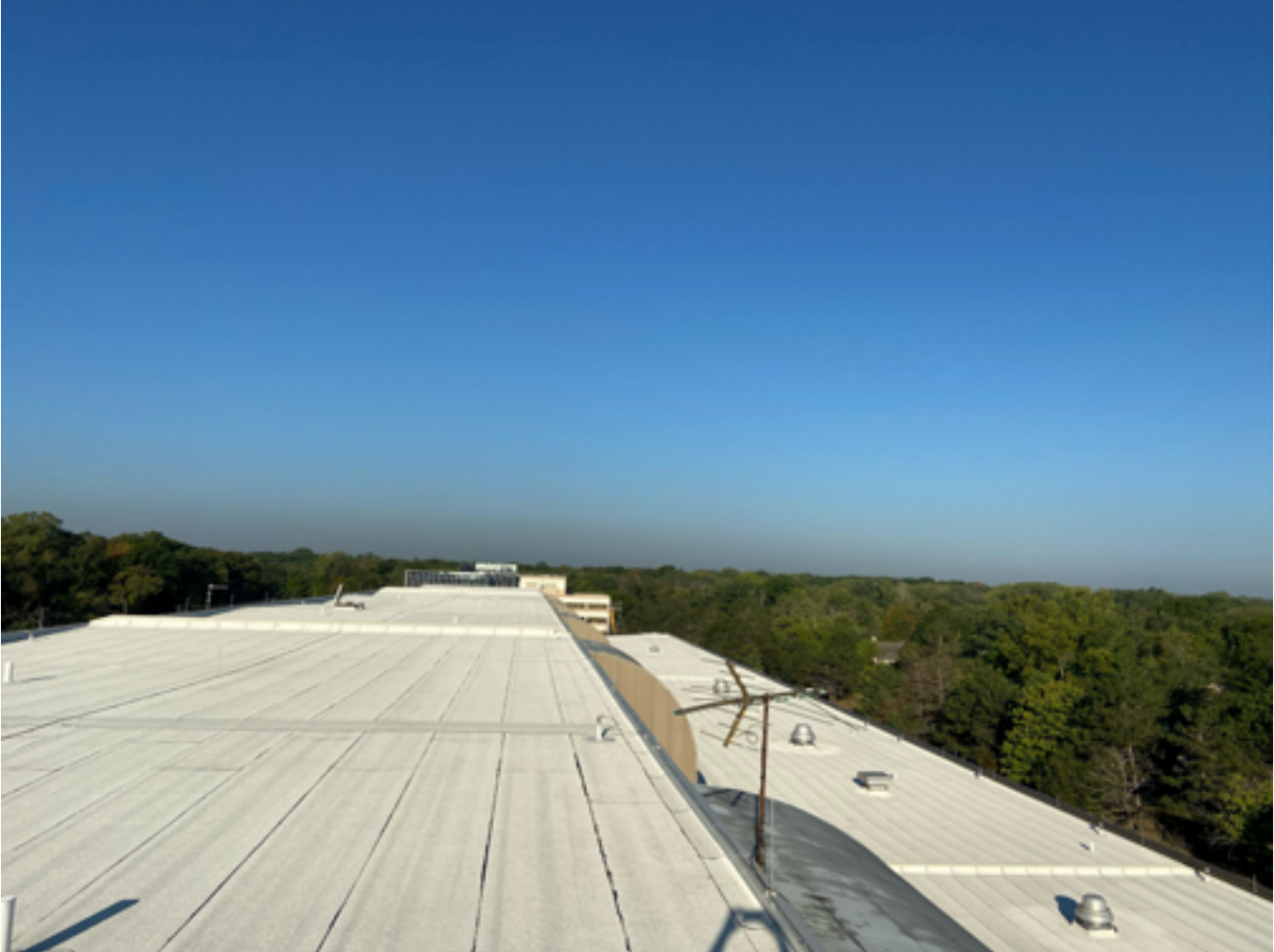
Roof replacement on District 2 (Skokie) courthouse
