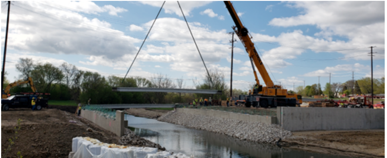
Figure 10: Bridges are large and complex structures and proper maintenance of County bridges is paramount to their safety and longevity.
