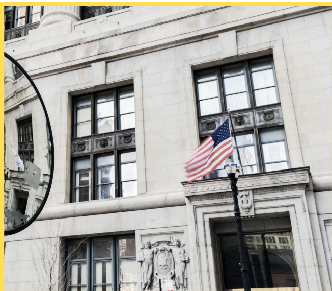
United States flag hangs outside of Cook County Central Building.
