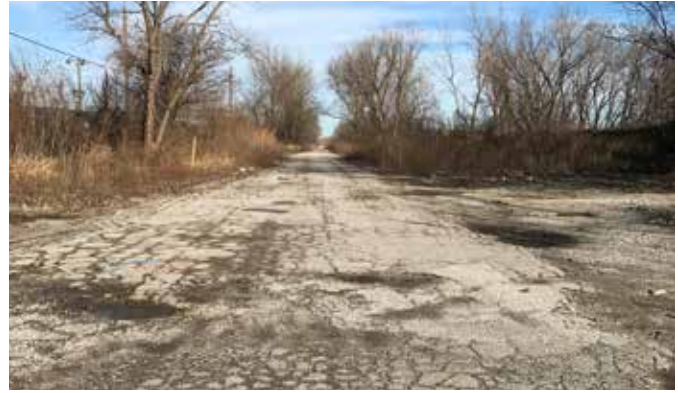
Poor pavement conditions on Stony Island Avenue between 122nd Street and the Calumet River/Lake Calumet in the City of Chicago.
